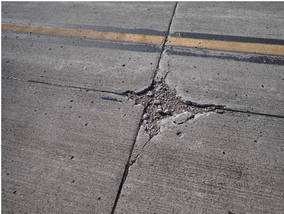
T01EG-02. ASR (Sample Unit No. 03).
