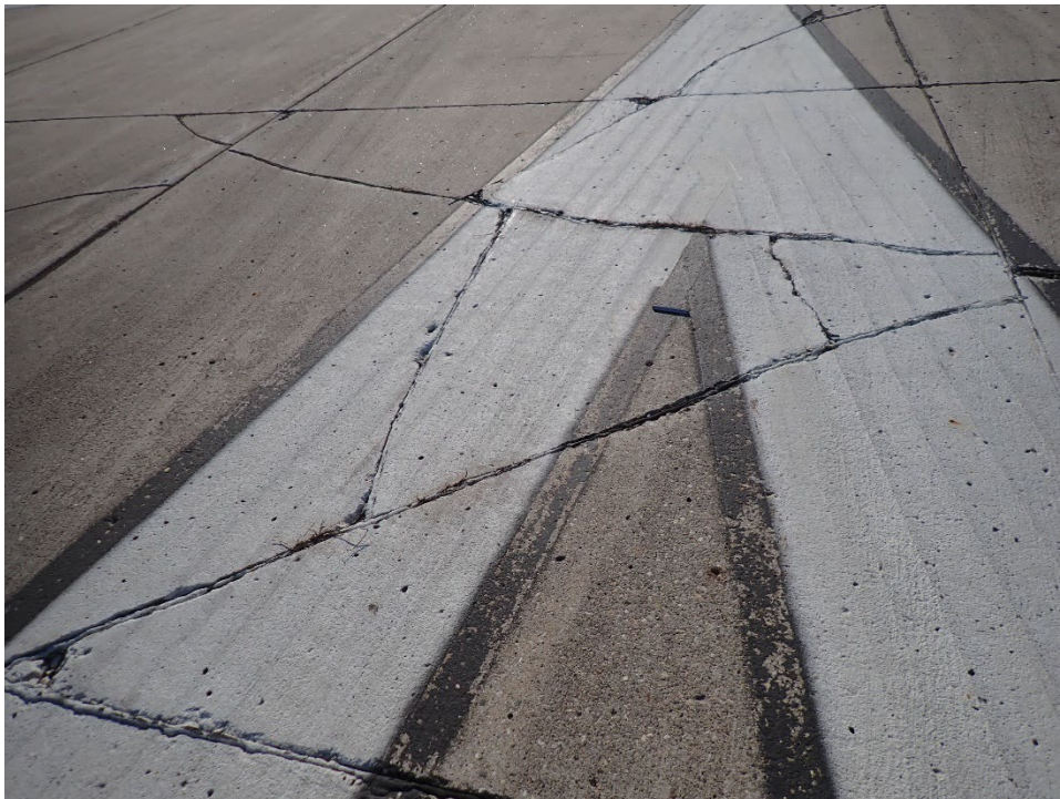
R13EG-01. Shattered Slab (Sample Unit No. 04).
