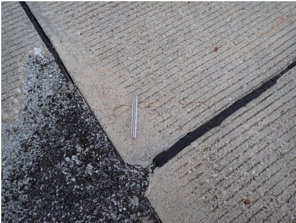
R12DN-01. ASR (Additional Sample Unit No. 36).
