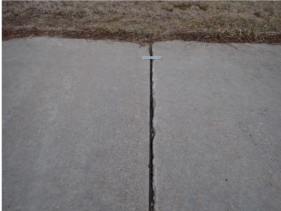
T01DN-04. Faulting (Sample Unit No. 01).
