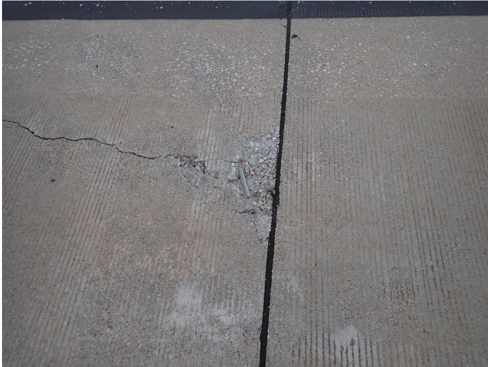
R12DN-02. ASR (Additional Sample Unit No. 15).
