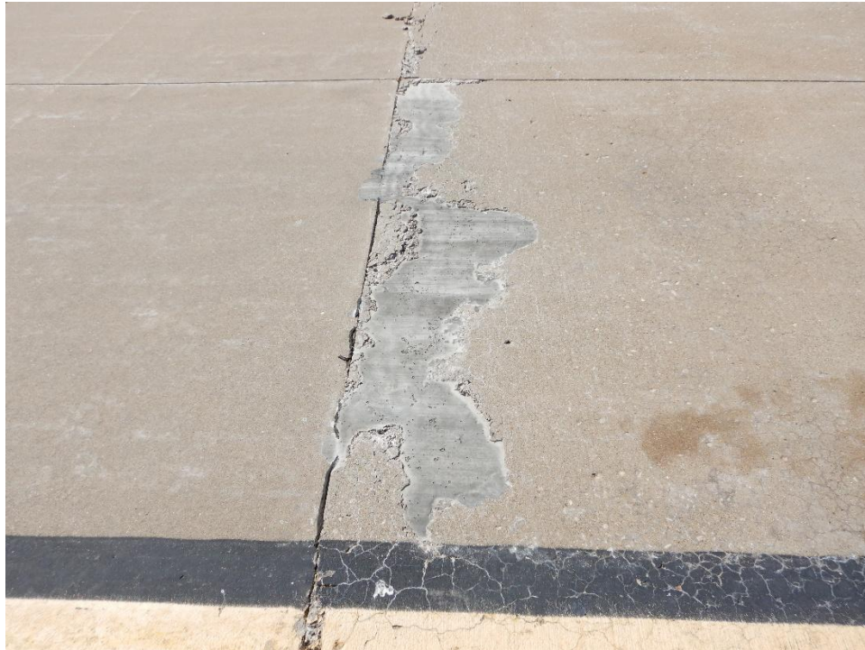
TB1DA-01. Large Patching (Sample Unit No. 01).
