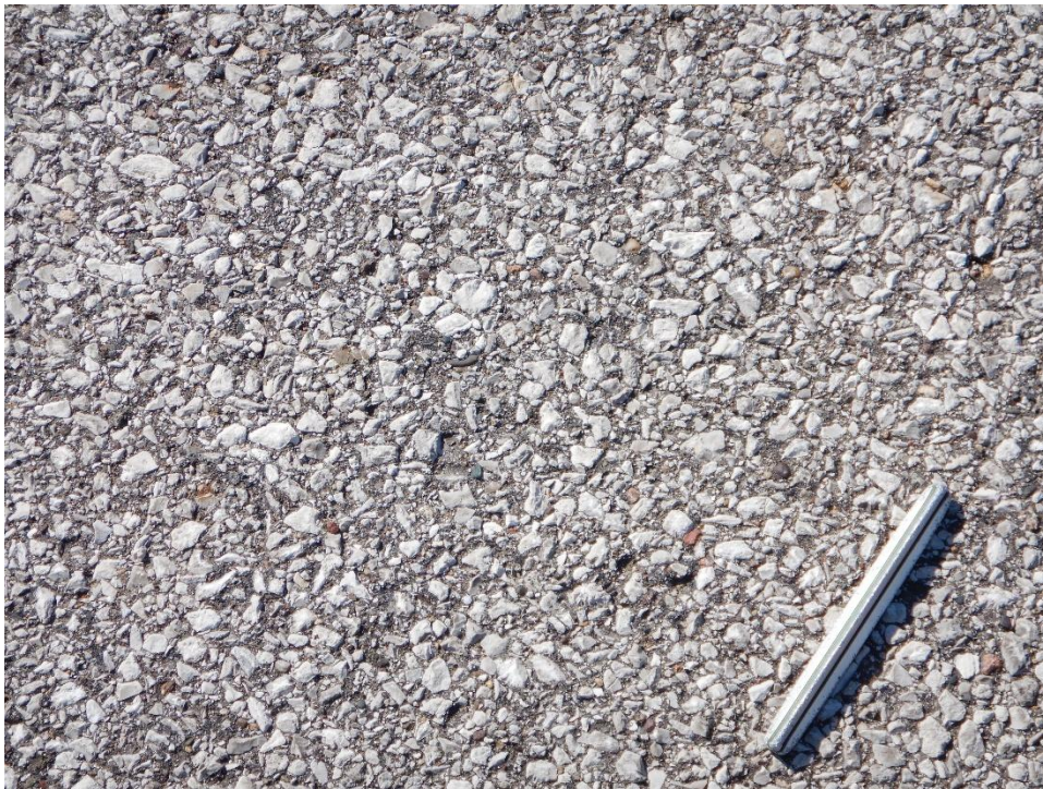
TH01DA-02. Weathering (Sample Unit No. 05).
