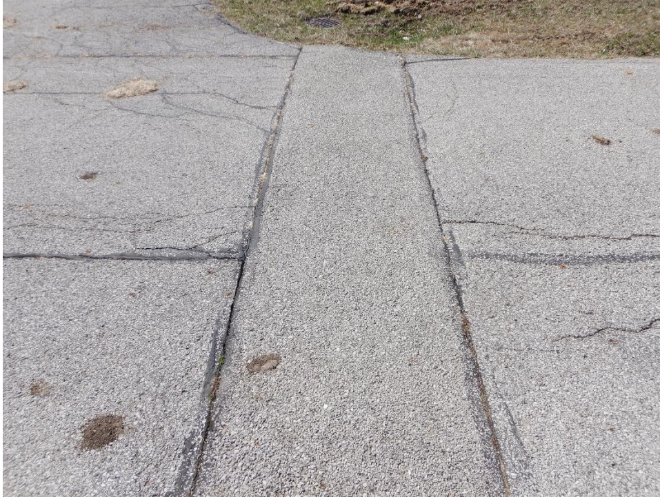
TH01DA-02. Patching (Sample Unit No. 05).
