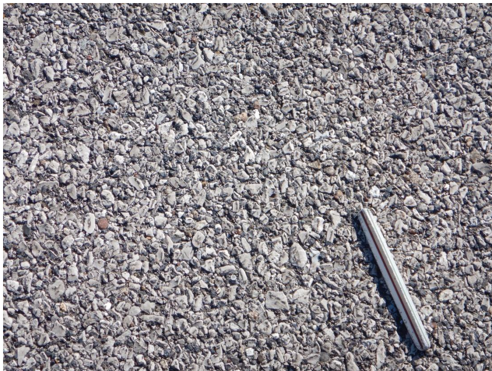
TH01DA-01. Weathering (Sample Unit No. 02).
