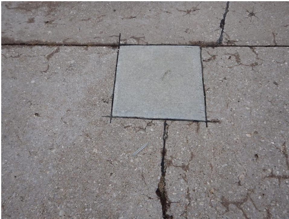
A01DA-01. Small Patching (Sample Unit No. 07).
