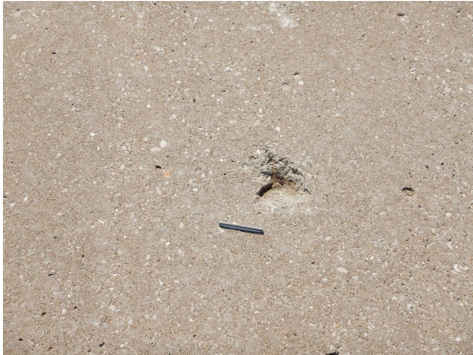
TADA-02. Scaling (Sample Unit No. 04).
