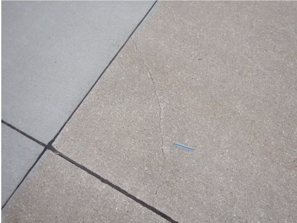
T01CT-01. Corner Break (Sample Unit No. 01).
