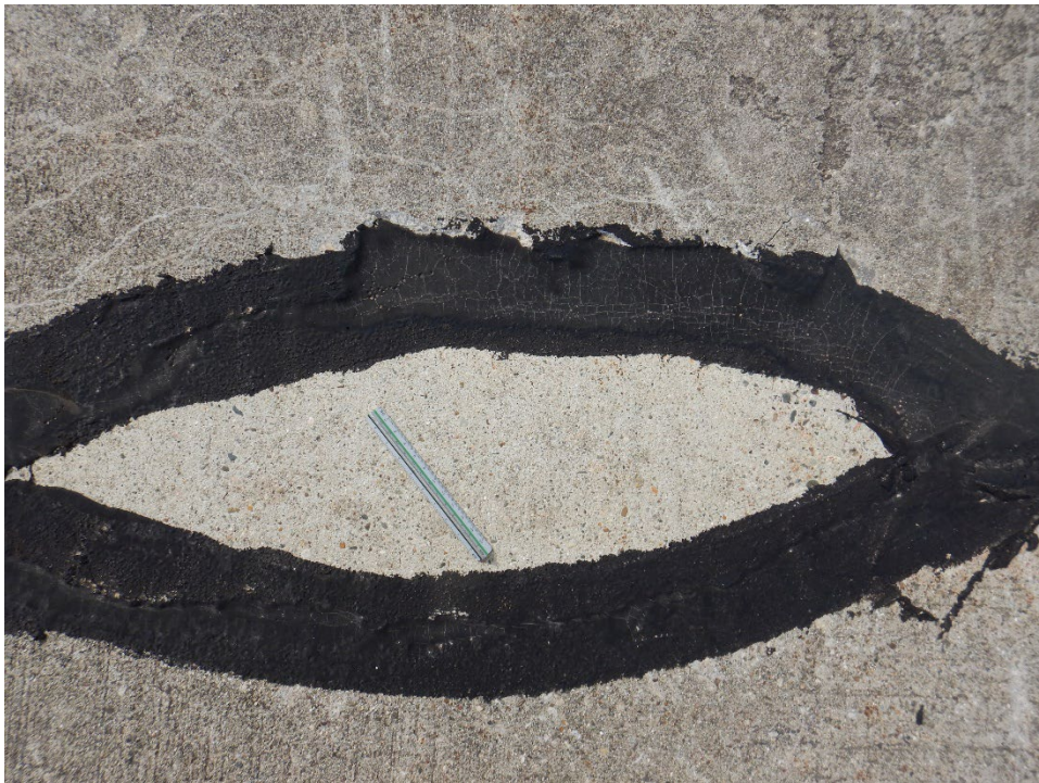
R15CR-02. Small Patching (Sample Unit No. 01).
