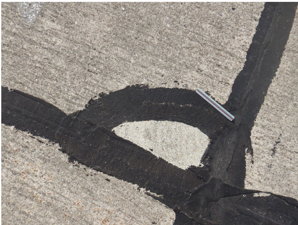
R15CR-01. Small Patching (Sample Unit No. 04).
