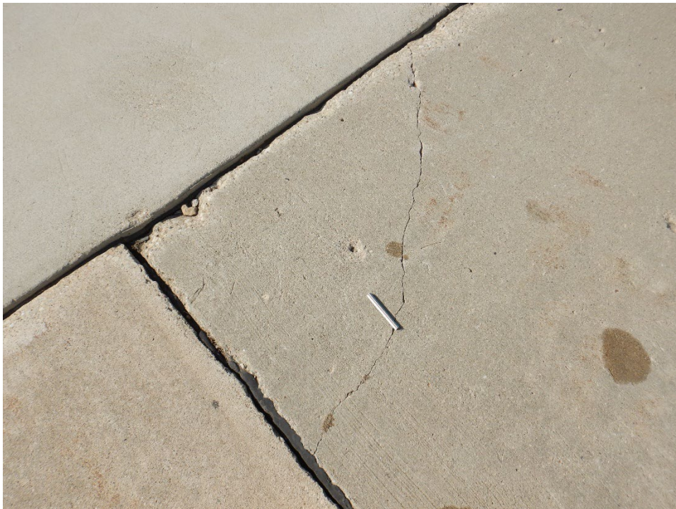
A02CR-02. Corner Break (Sample Unit No. 01).
