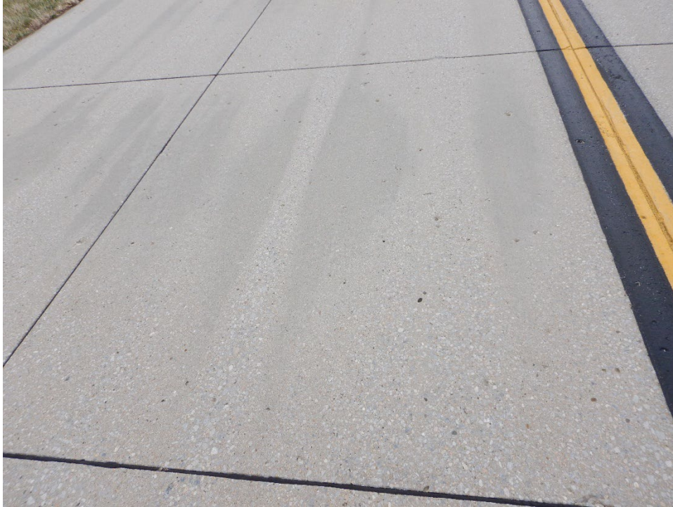
TCCB-02. Popouts (Sample Unit No. 17).
