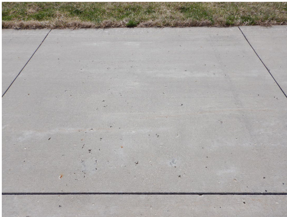
TACB-01. Popouts (Sample Unit No. 15).
