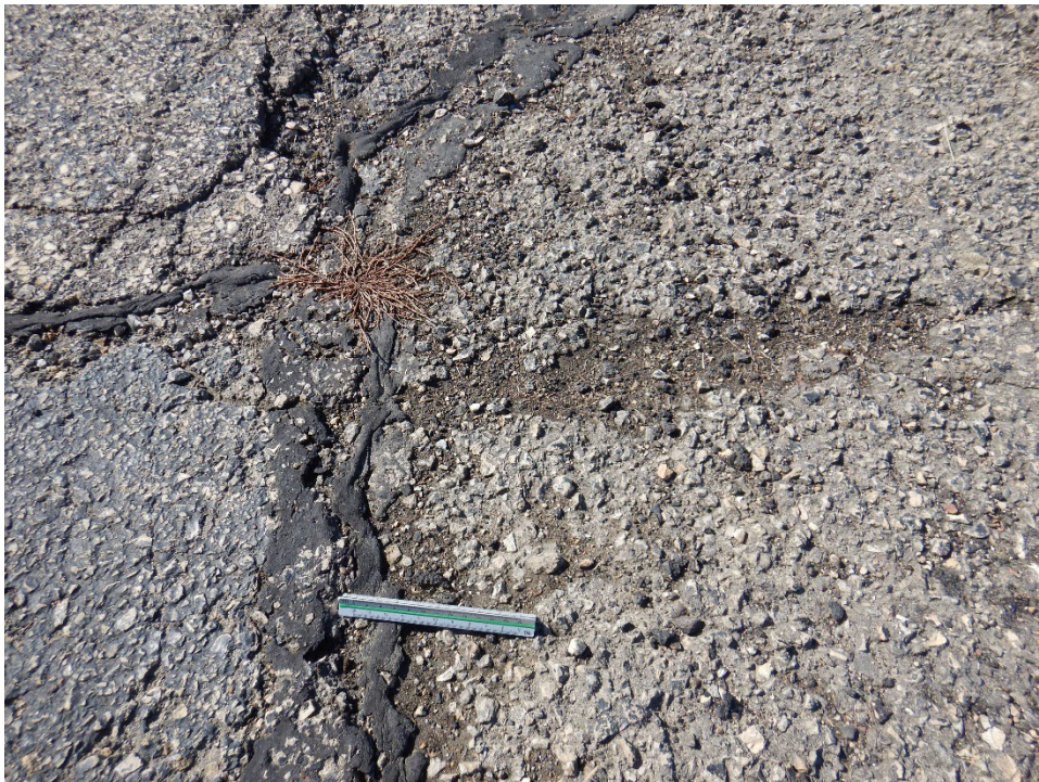
T04CN-01. Raveling (Sample Unit No. 01).
