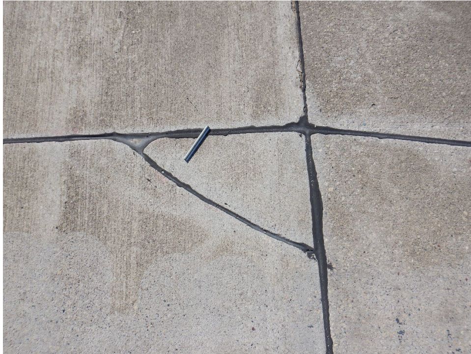
TACN-02. Corner Break (Sample Unit No. 01).
