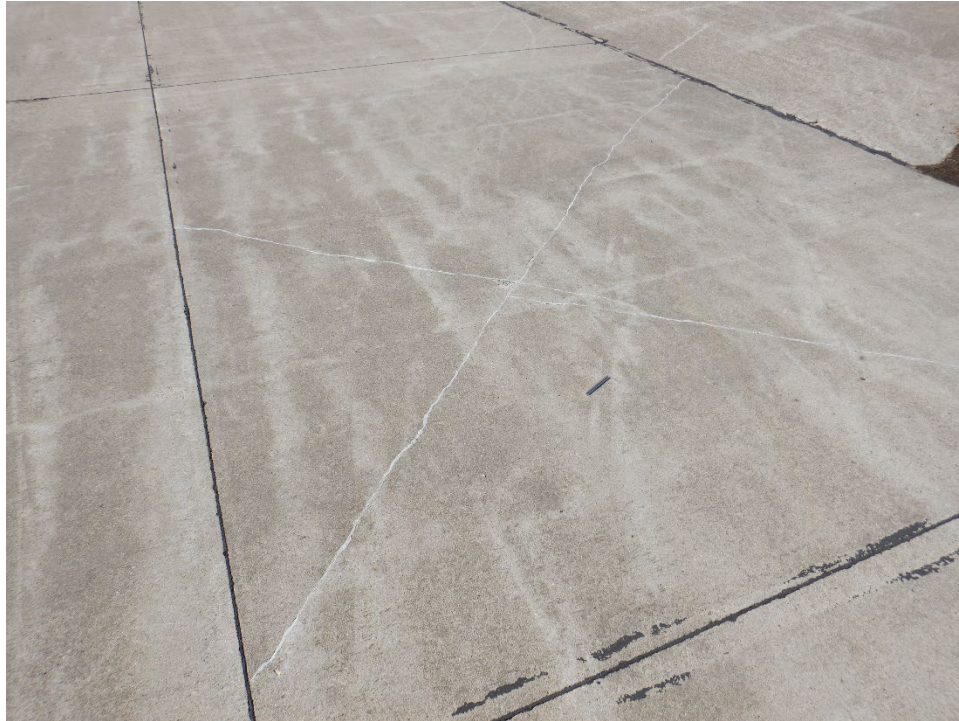
TH01CN-02. Shattered Slab (Sample Unit No. 01) (1).
