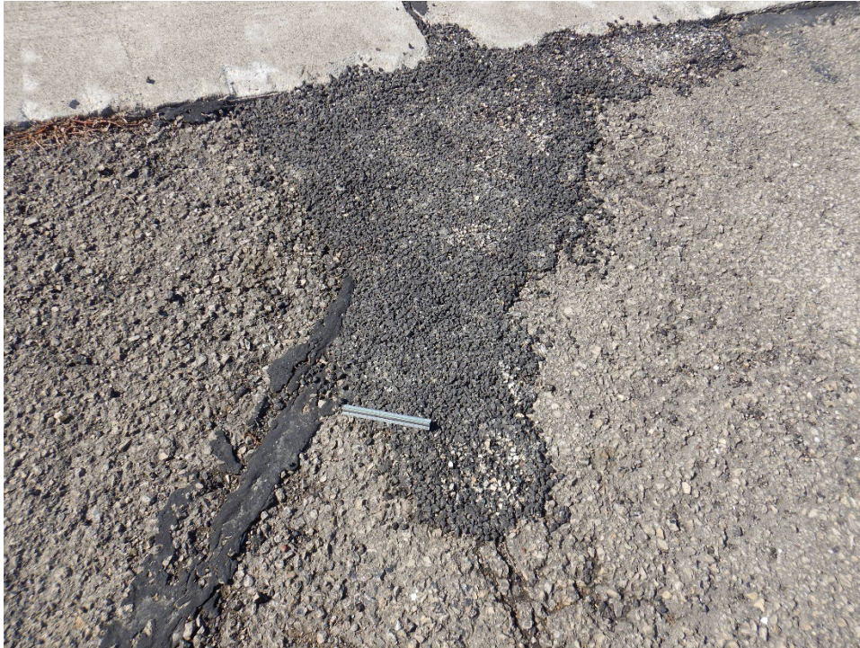
T04CN-01. Patching (Sample Unit No. 01).
