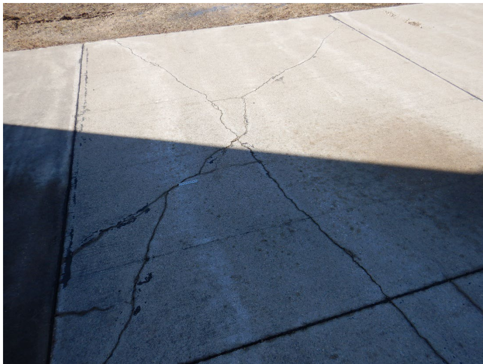
TH01CN-02. Shattered Slab (Sample Unit No. 01) (2).
