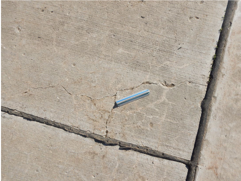
T01CD-01. ASR (Sample Unit No. 07).
