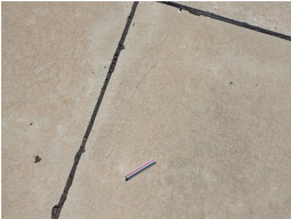
T02CD-01. ASR (Sample Unit No. 06).
