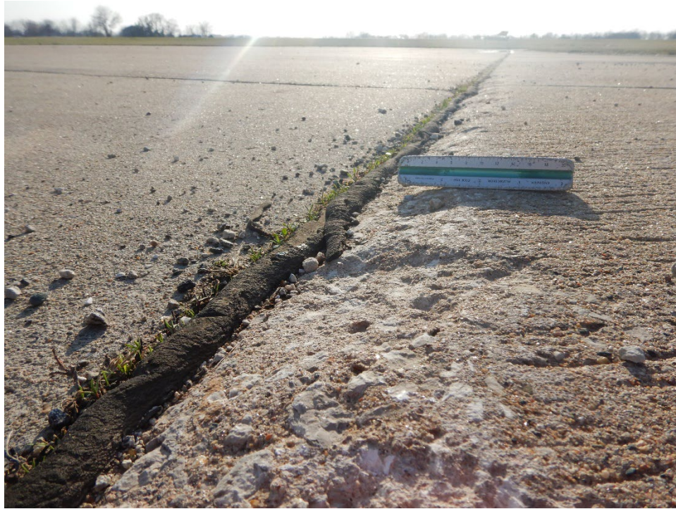
T02CH-01. Faulting (Sample Unit No. 001).
