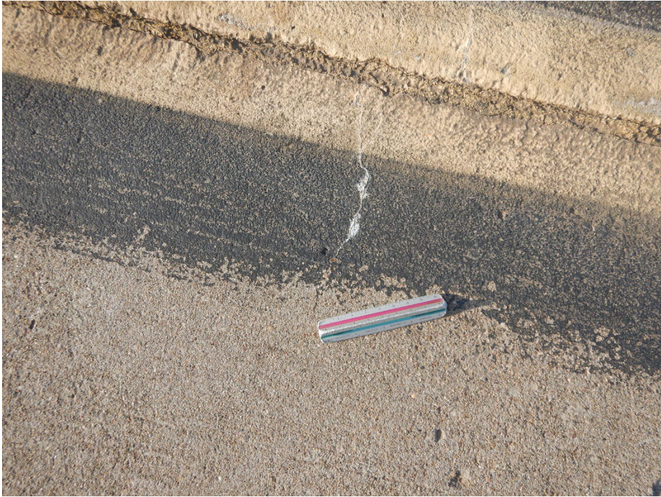
A02CH-01. ASR (Sample Unit No. 011).
