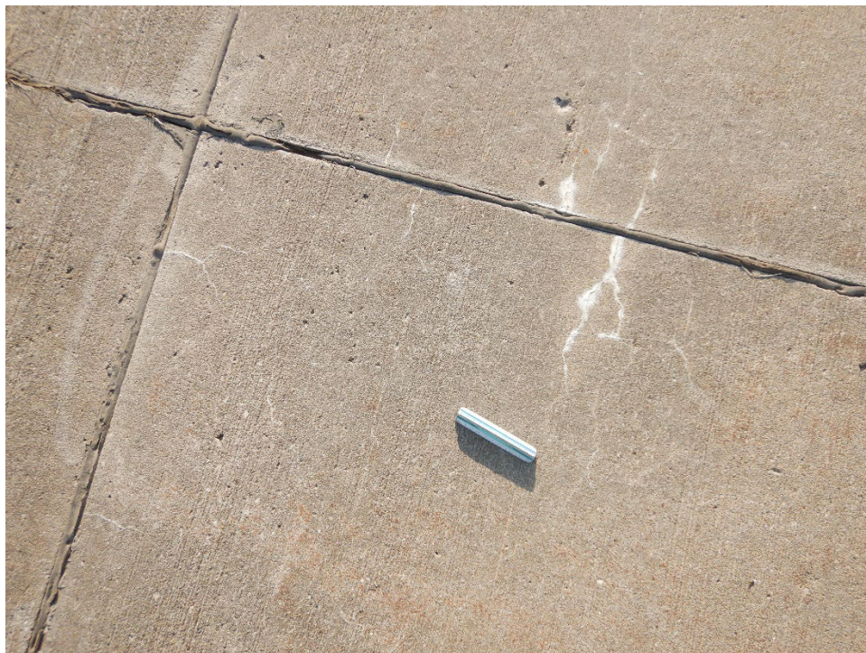
A02CH-01. ASR (Sample Unit No. 007).
