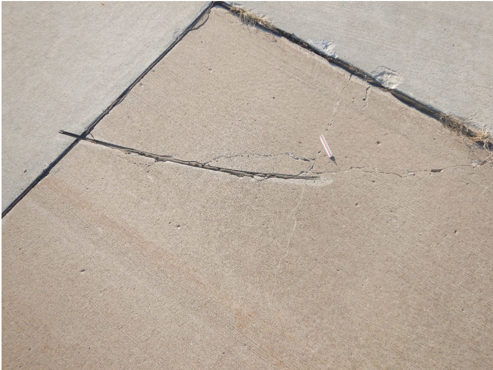
T02CH-01. Corner Break (Sample Unit No. 005).
