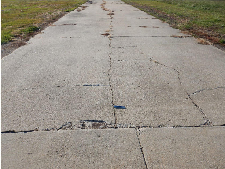
TH01CH-02. Shattered Slab (Sample Unit No. 01).
