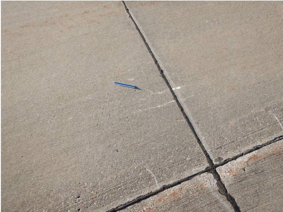
T03CH-01. ASR (Sample Unit No. 07).
