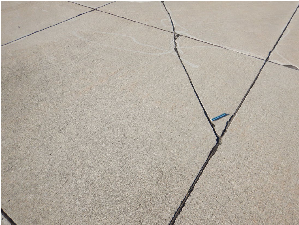
A01CH-01. Corner Break (Additional Sample Unit No. 11).
