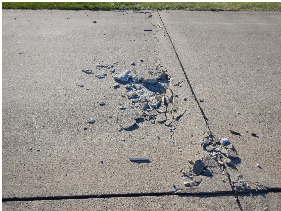
R16CE-03. Blow-Up (Additional Sample Unit No. 07).
