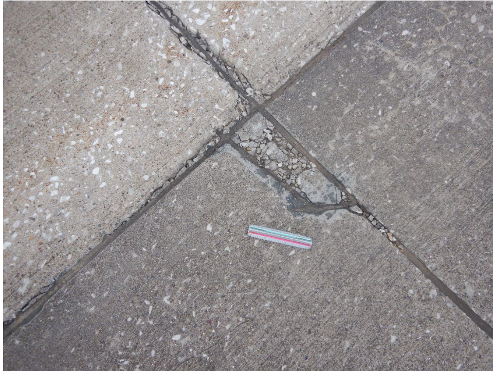
TA3BR-01. Small Patching (Sample Unit No. 03).
