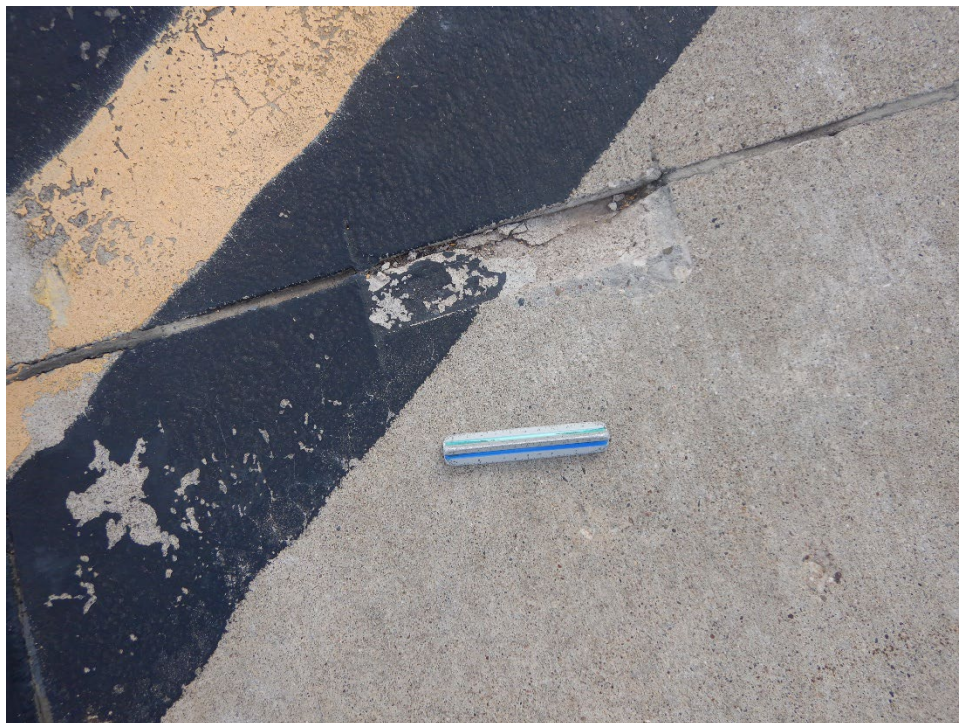
TA2BR-01. Small Patching (Sample Unit No. 04).
