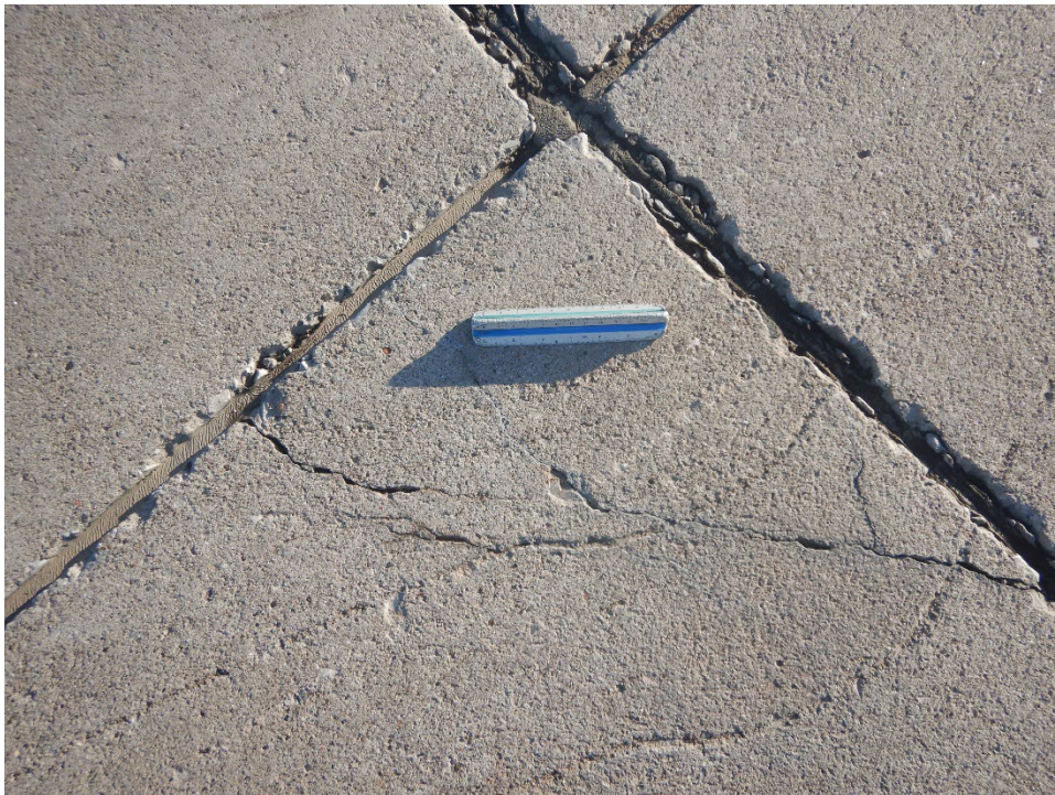
TCBR-01. ASR (Additional Sample Unit No. 11).
