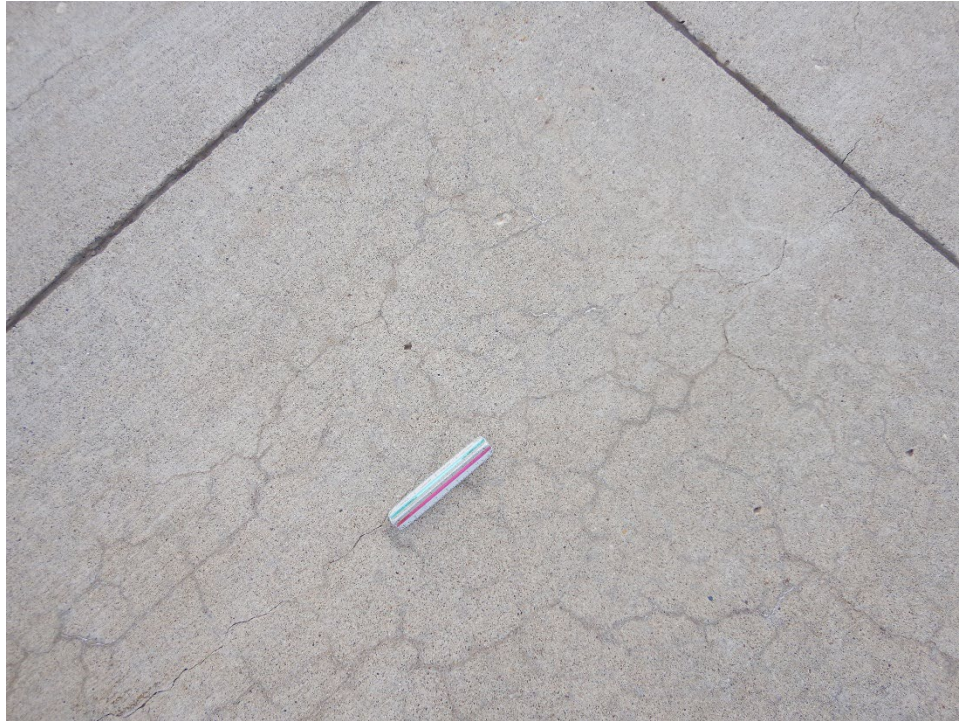
TA2BR-01. ASR (Sample Unit No. 04).
