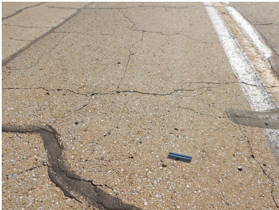
TDBR-04. Raveling (Sample Unit No. 02).
