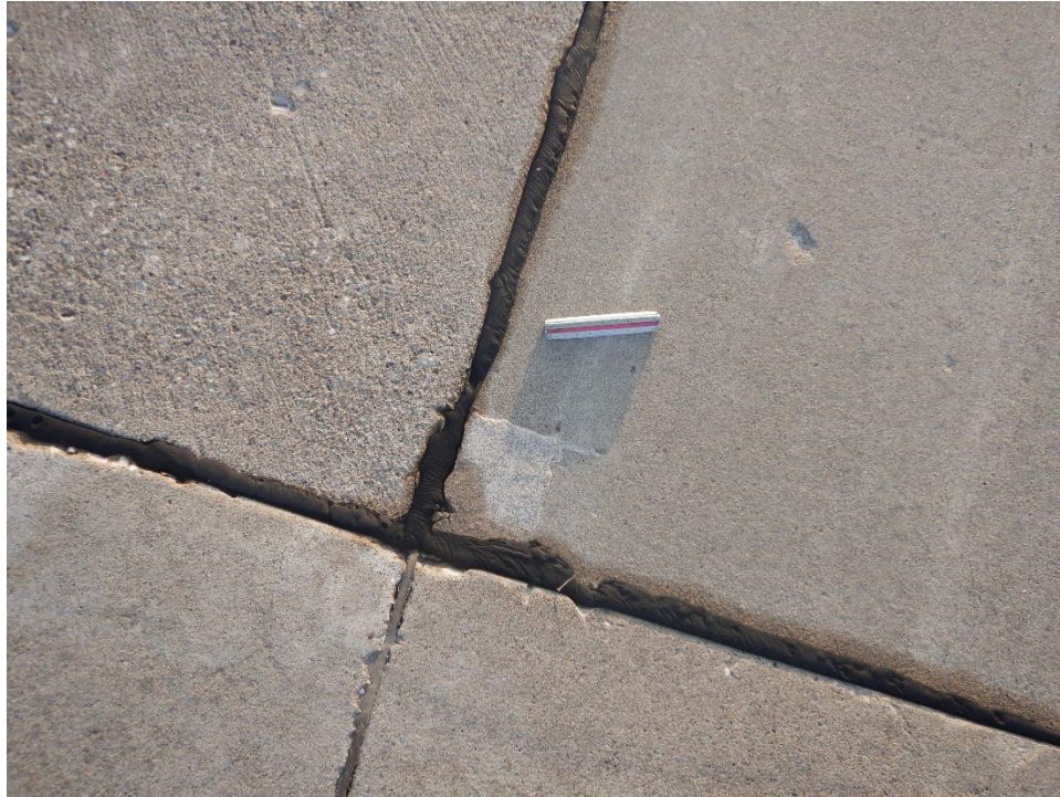
TA2BR-02. Small Patching (Sample Unit No. 05).
