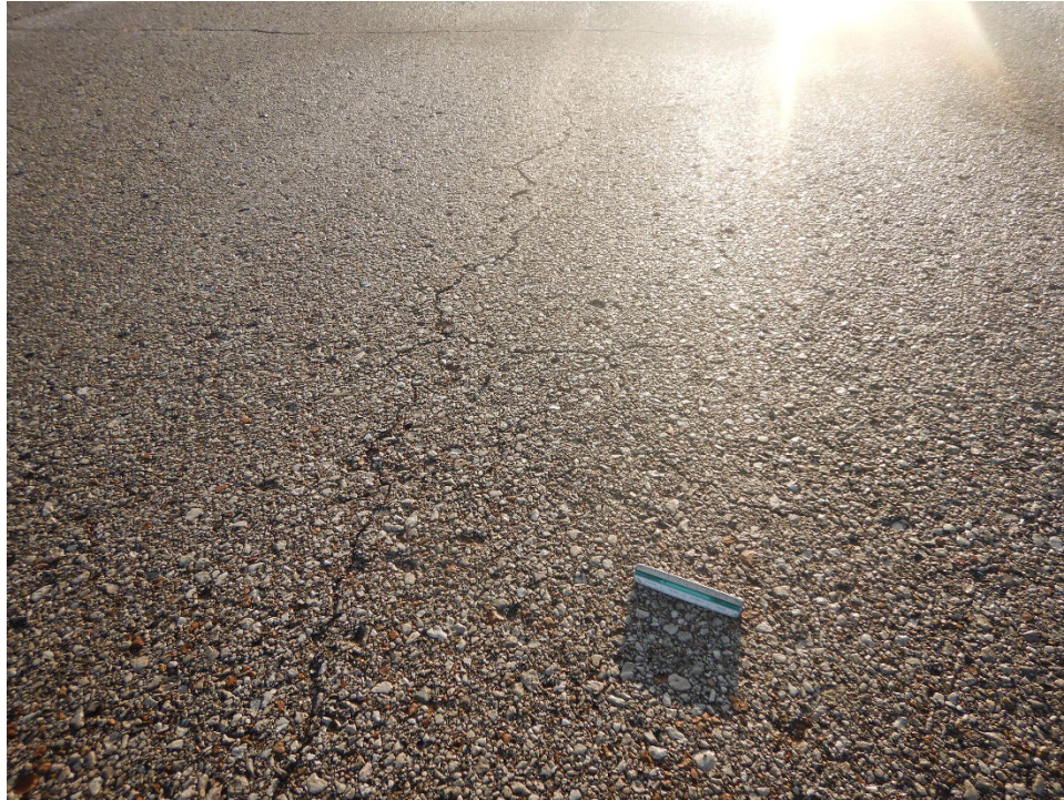
TH01BR-01. Raveling (Sample Unit No. 02).
