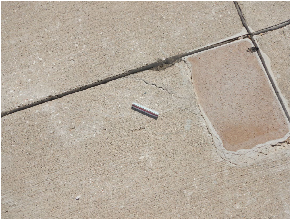
TABR-02. ASR (Sample Unit No. 94).
