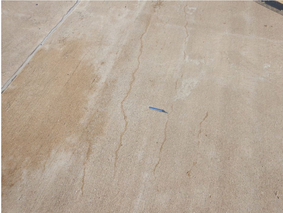
TCBR-01. ASR (Sample Unit No. 03).
