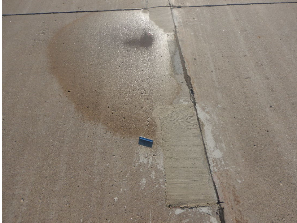
TCBR-01. Small Patching (Sample Unit No. 08).
