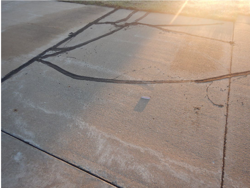
TH01BR-02. Shattered Slab (Additional Sample Unit No. 01).
