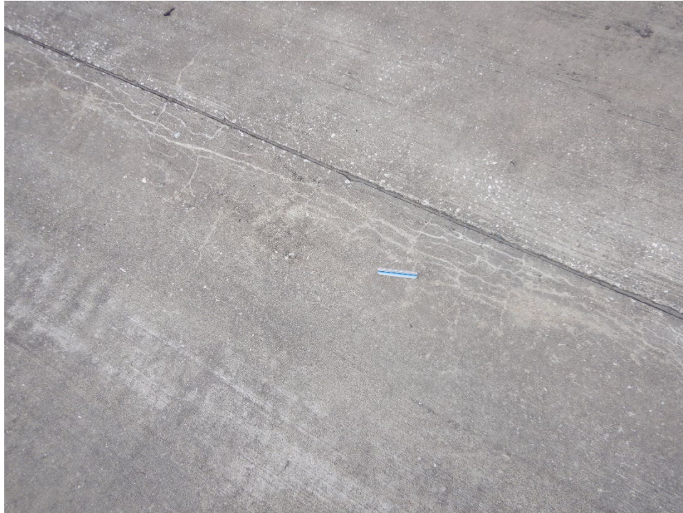
TA3BR-01. ASR (Sample Unit No. 02).
