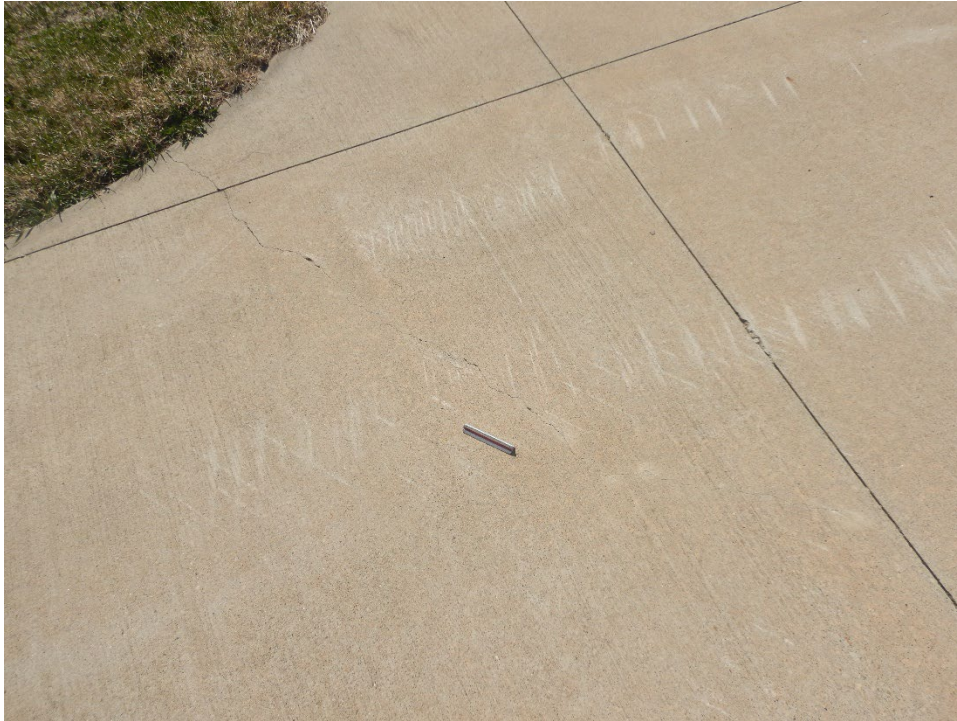
TH01BL-02. Corner Break (Sample Unit No. 01).
