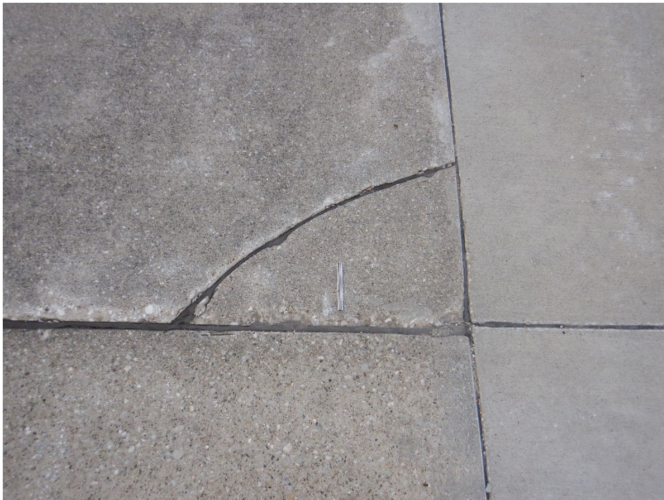
TH01BP-01. Corner Break (Sample Unit No. 01).
