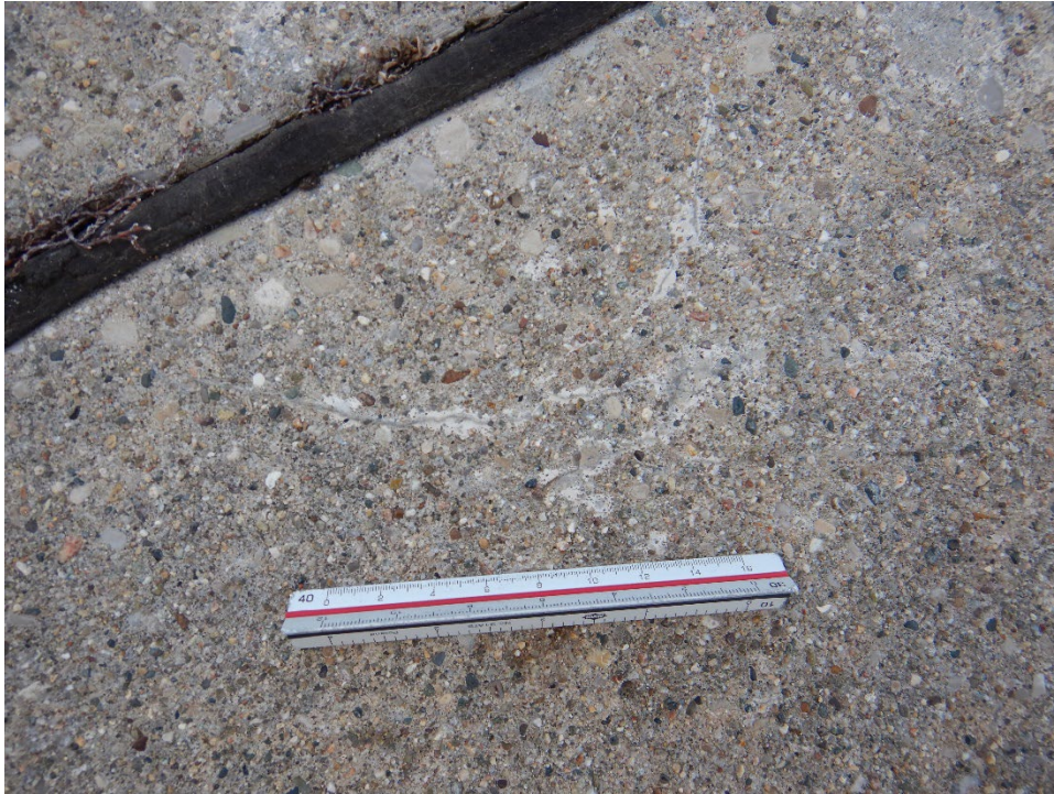
TH01BP-01. ASR (Sample Unit No. 01).
