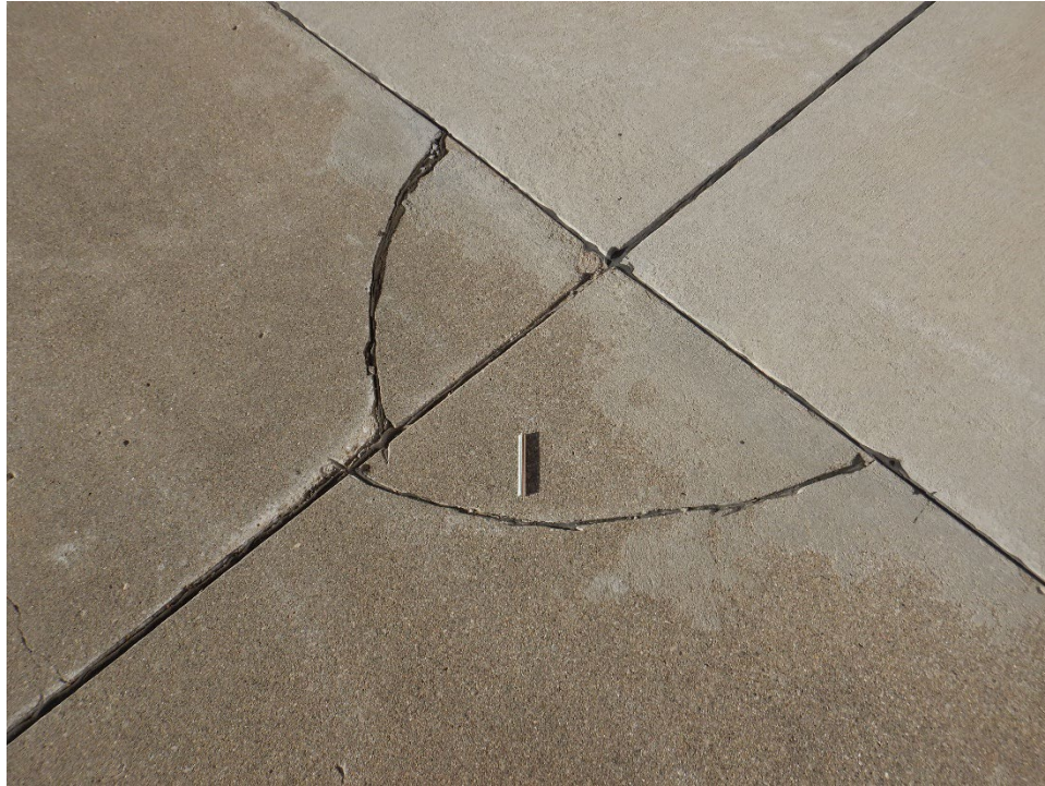
TH01BP-02. Corner Break (Sample Unit No. 01).
