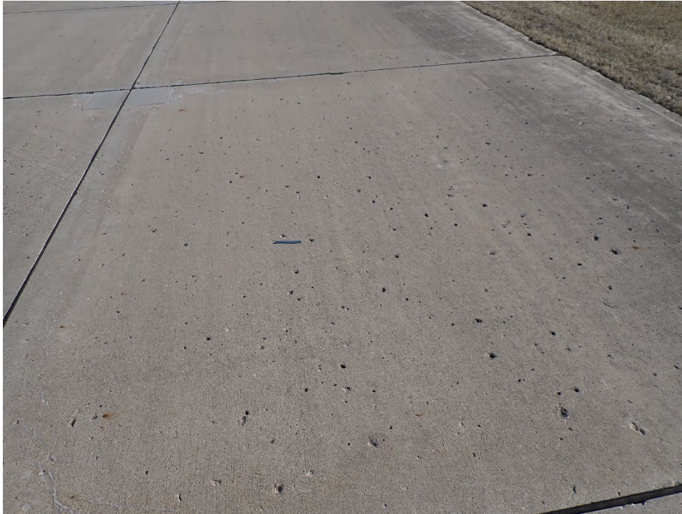
R04AN-02. Popouts (Sample Unit No. 03).
