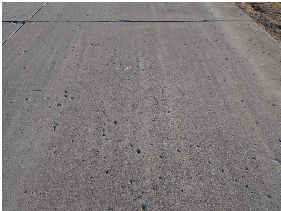
R04AN-03. Popouts (Sample Unit No. 05).
