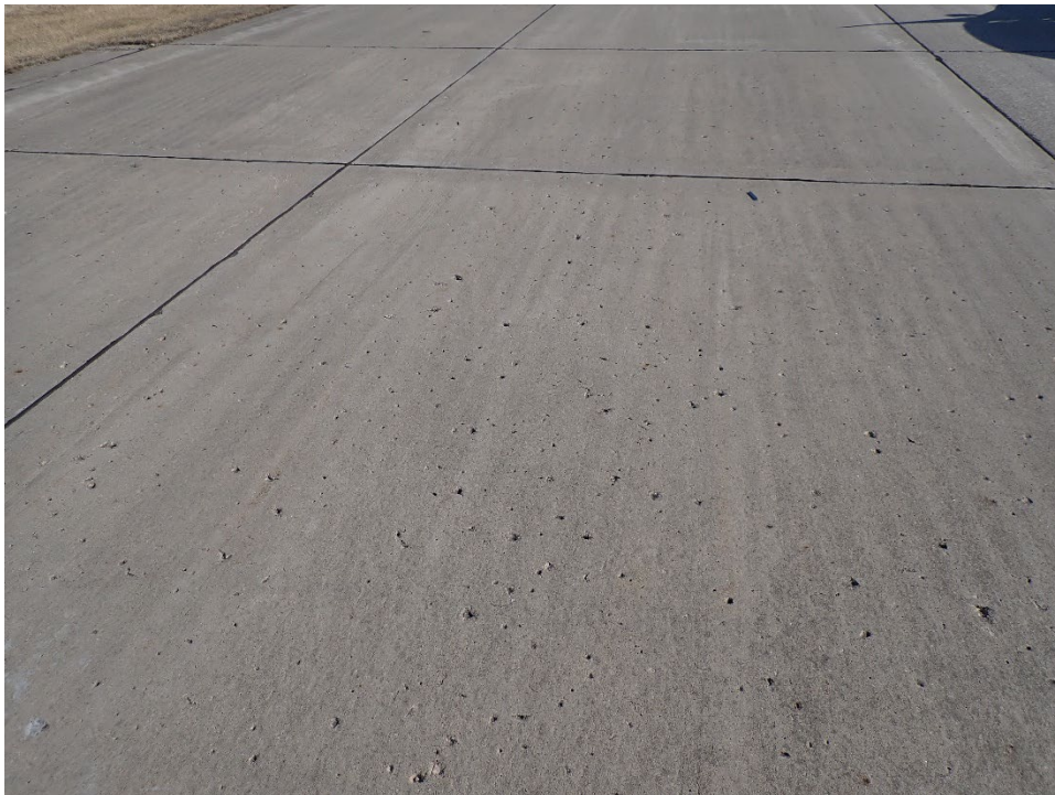
R04AN-02. Popouts (Sample Unit No. 04).
