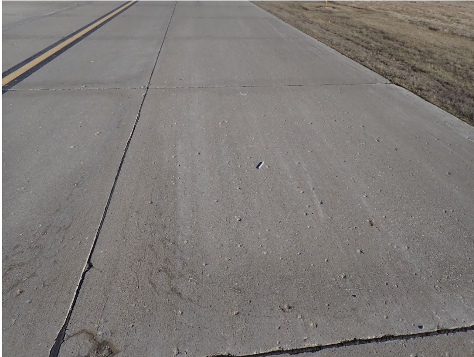
T02AN-01. Popouts (Sample Unit No. 06).
