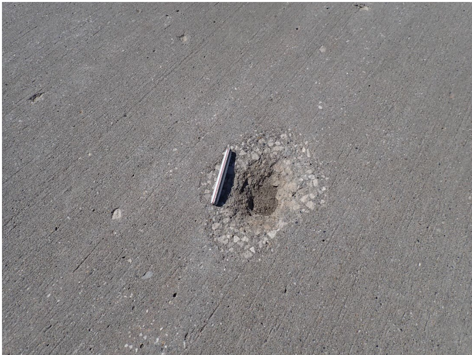
T07AN-01. Small Patching (Sample Unit No. 04).
