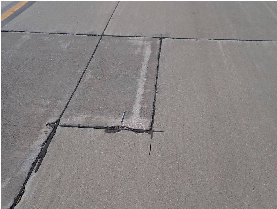
T12AN-01. Large Patching (Sample Unit No. 18).
