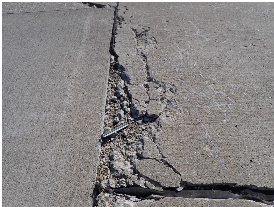
R18AN-01. ASR (Sample Unit No. 63).
