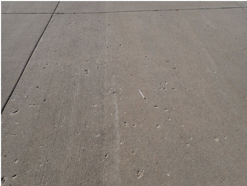
TH01AN-01. Popouts (Sample Unit No. 04).
