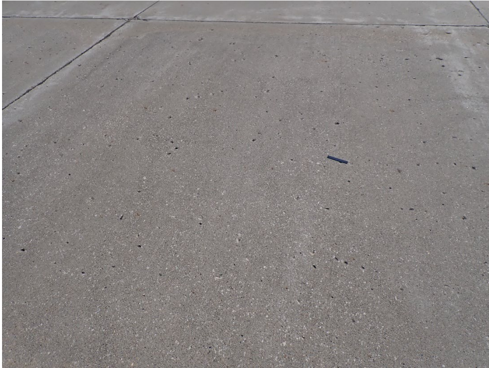
A01AN-02. Popouts (Sample Unit No. 05).
