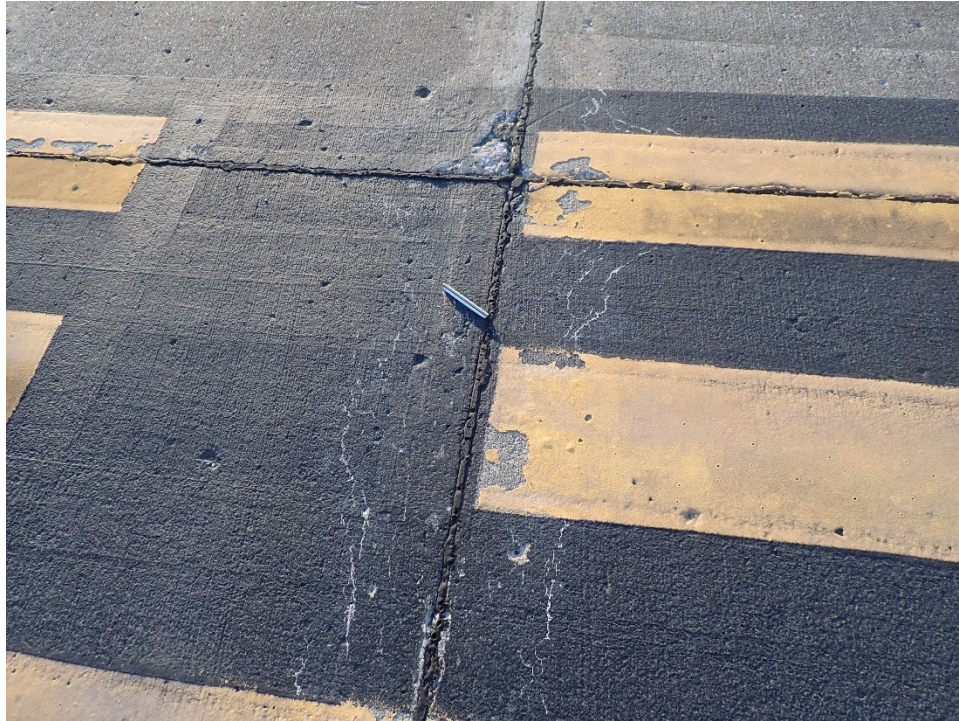
T09AN-01. ASR (Sample Unit No. 02).
