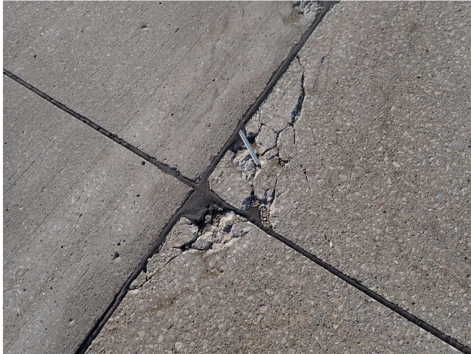
T02AN-01. ASR (Sample Unit No. 03).
