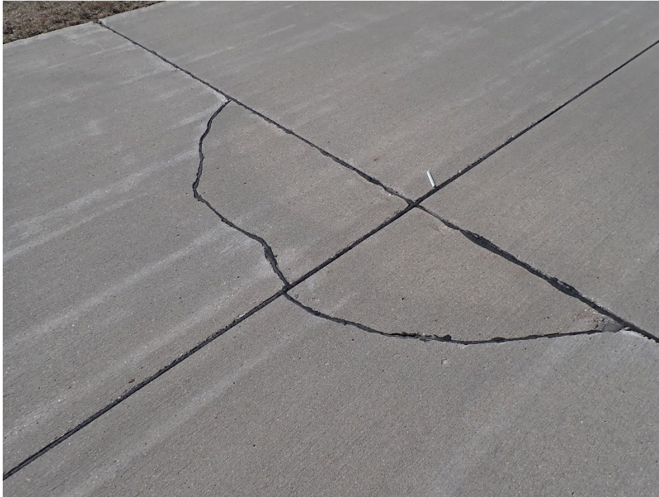
T07AN-01. Corner Break (Sample Unit No. 04).
