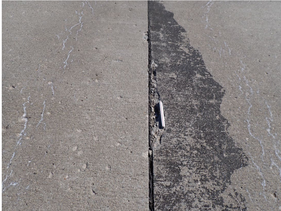
T05AN-01. ASR (Sample Unit No. 01).
