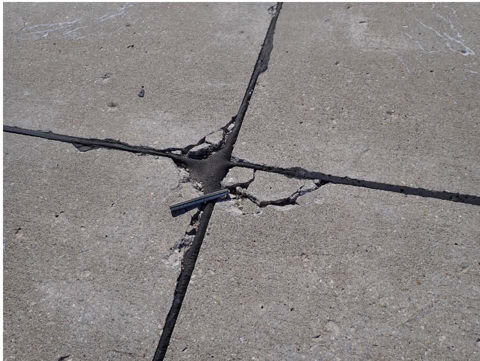
T05AN-01. ASR (Sample Unit No. 05).
