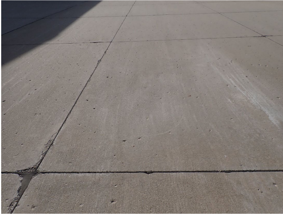
TH01AN-01. Popouts (Sample Unit No. 01).
