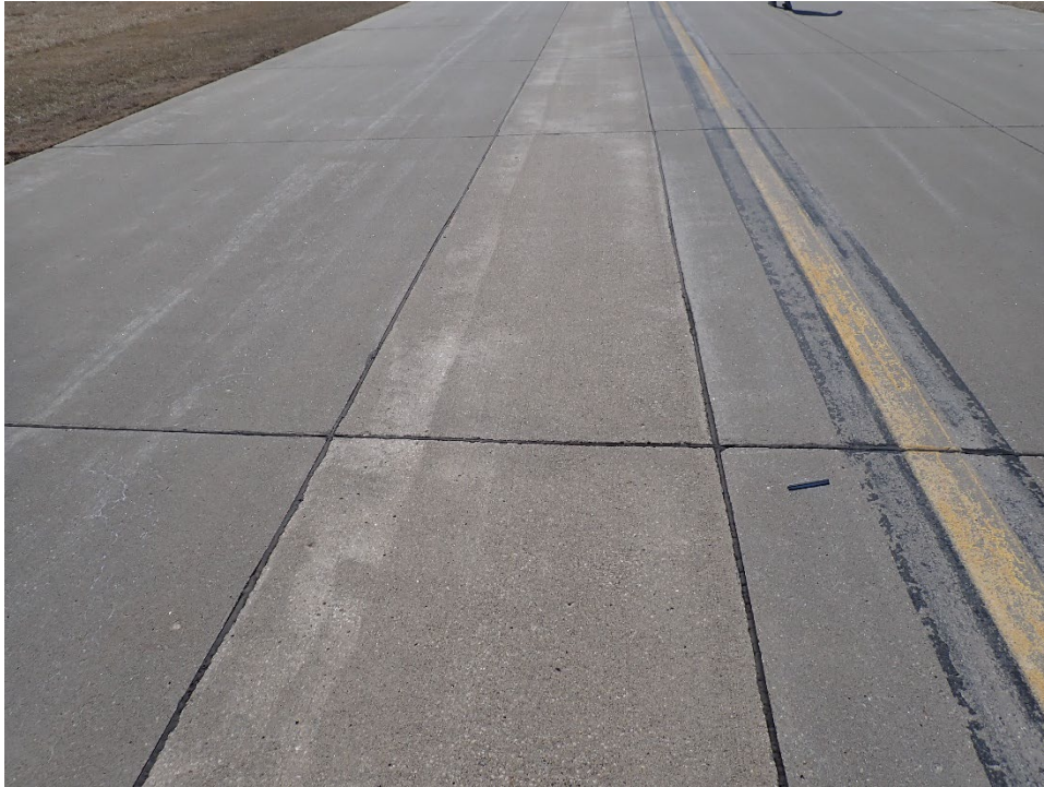
T06AN-01. Large Patching (Sample Unit No. 12).
