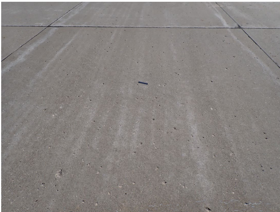
A01AN-01. Popouts (Sample Unit No. 33).
