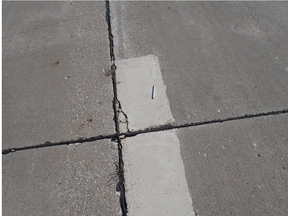
T08AN-01. Small Patching (Sample Unit No. 04).
