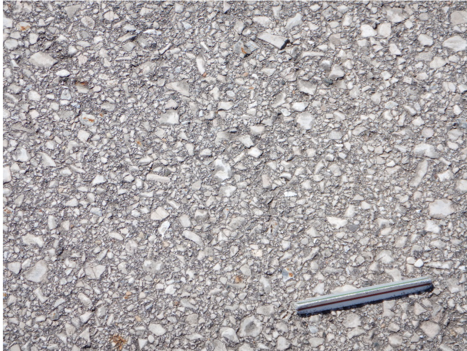
TBAM-01. Weathering (Sample Unit No. 07).
