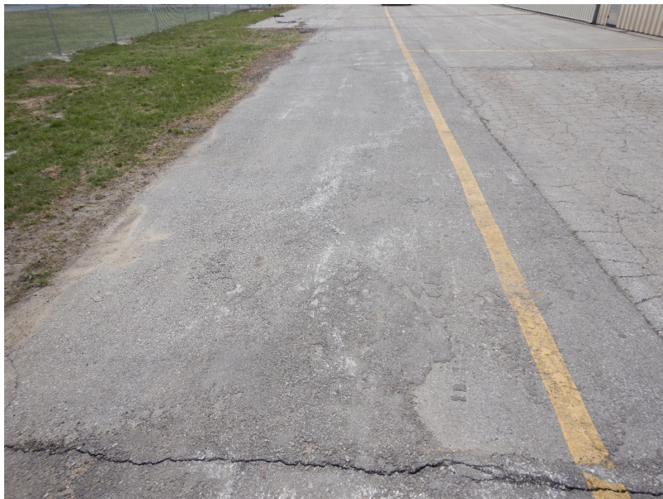
TH01AM-01. Patching (Sample Unit No. 02).
