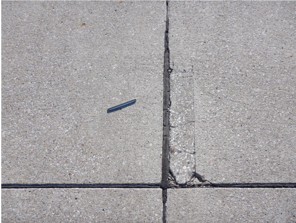
TAAM-06. Small Patching (Sample Unit No. 03).
