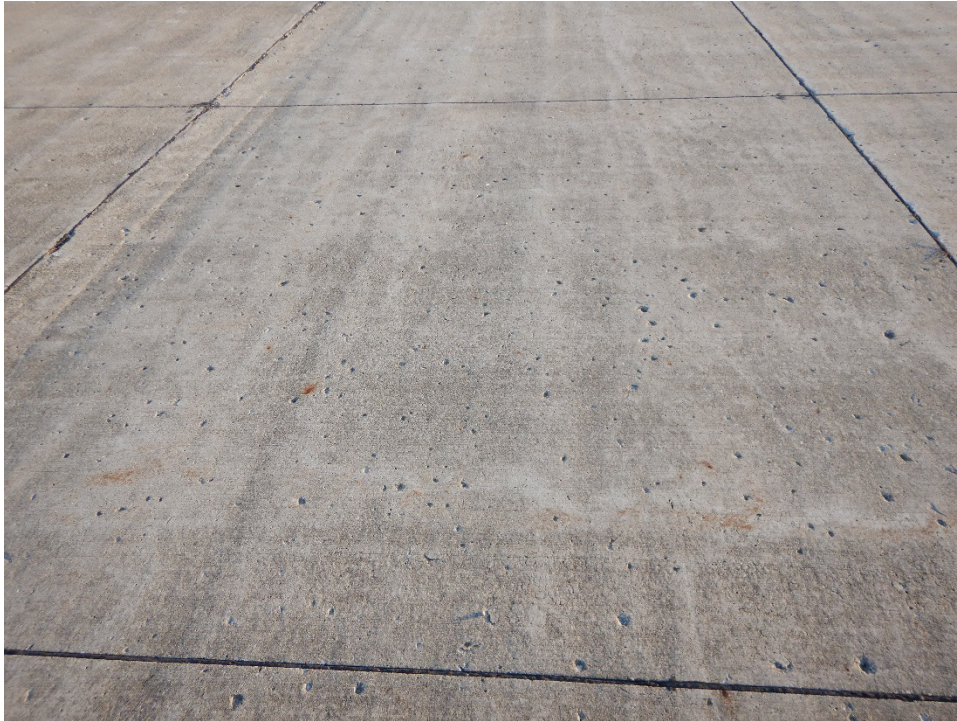
TAAM-10. Popouts (Sample Unit No. 04).
