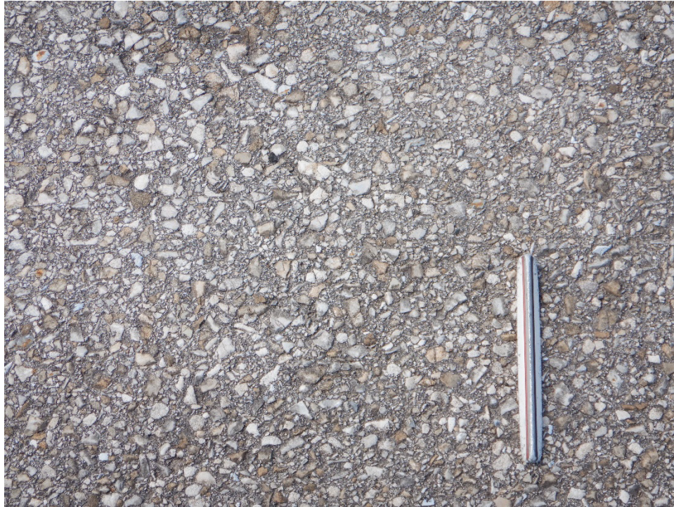
TBAM-03. Weathering (Sample Unit No. 01).
