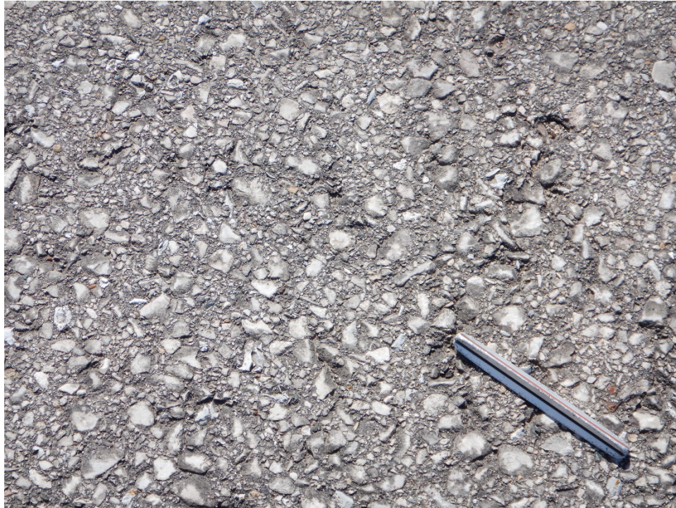
TB1AM-01. Weathering (Sample Unit No. 02).
