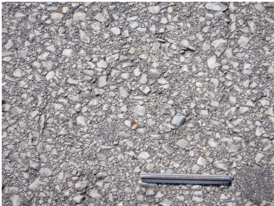
TBAM-01. Weathering (Sample Unit No. 09).
