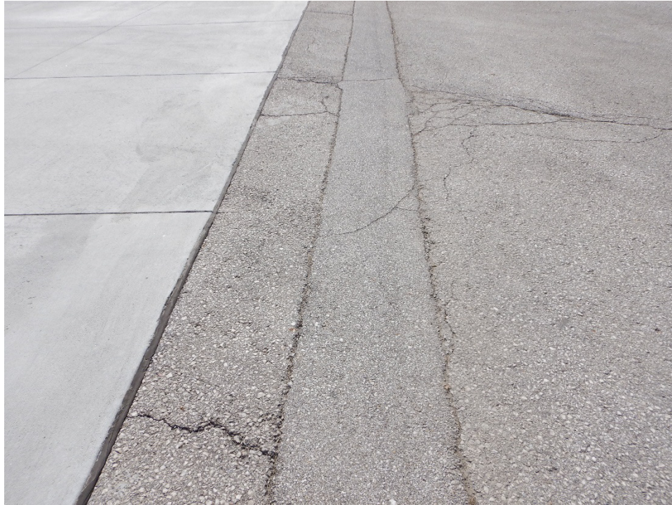
TA1AM-02. Patching (Sample Unit No. 03).
