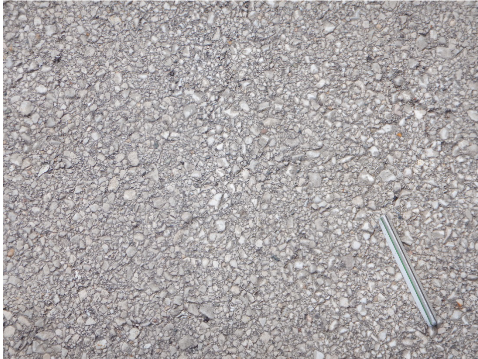
TH01AM-01. Weathering (Sample Unit No. 02).
