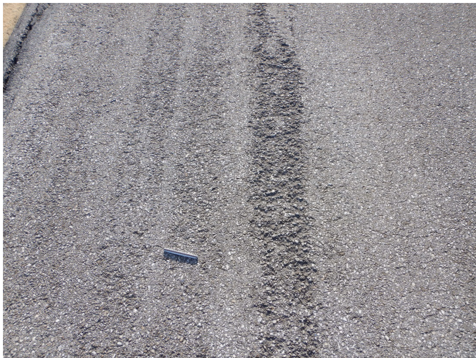
TA2AM-01. Raveling (Sample Unit No. 03).
