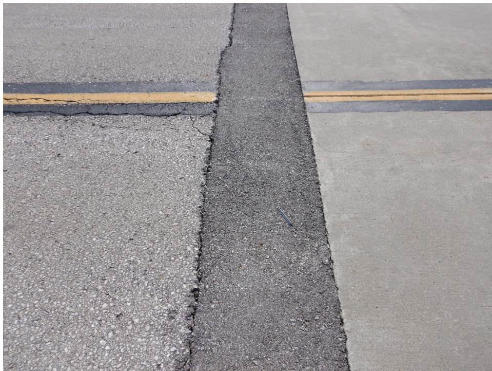
TB1AM-01. Patching (Sample Unit No. 02).
