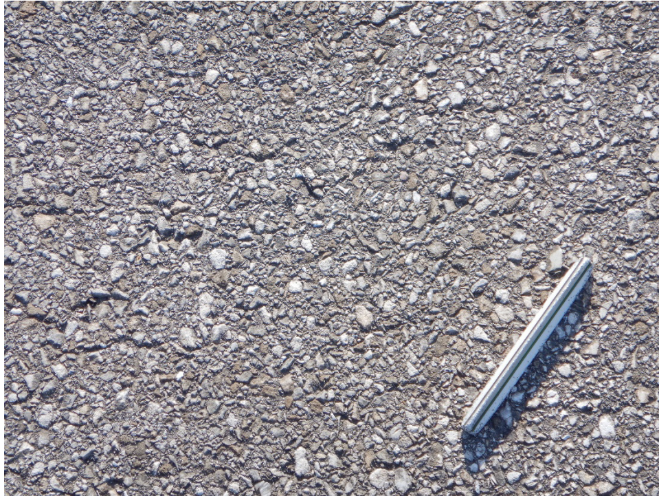
TA2AM-01. Weathering (Sample Unit No. 01).
