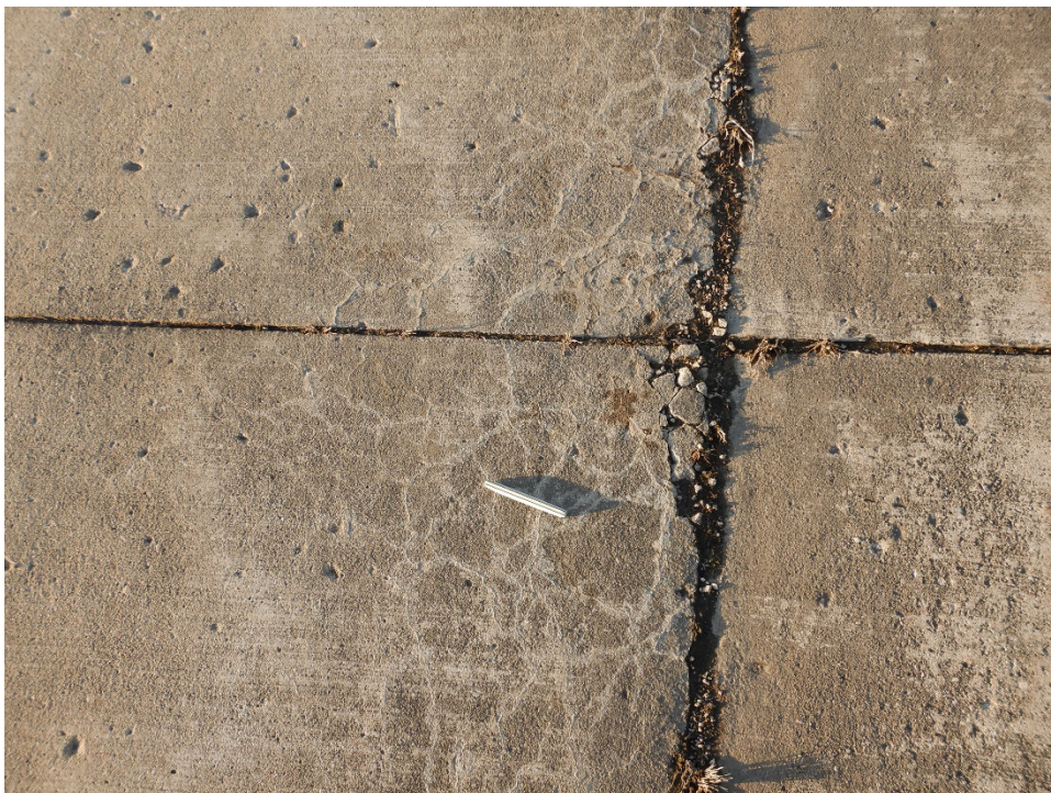
TAAM-10. ASR (Additional Sample Unit No. 07) (1).
