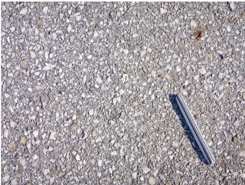
R13AM-02. Weathering (Sample Unit No. 04).
