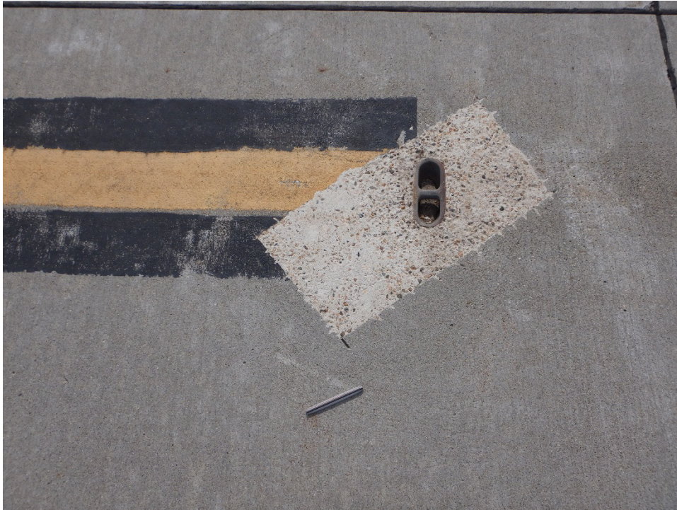
A01AM-02. Small Patching (Sample Unit No. 23).
