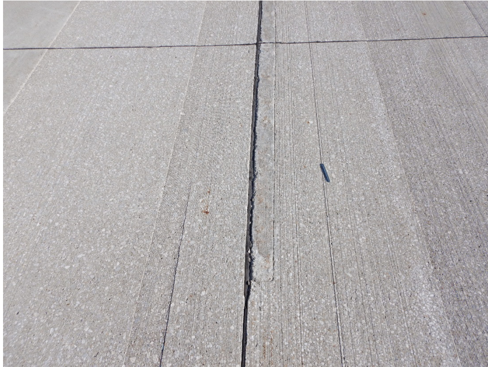
R13AM-01. Small Patching (Sample Unit No. 75).
