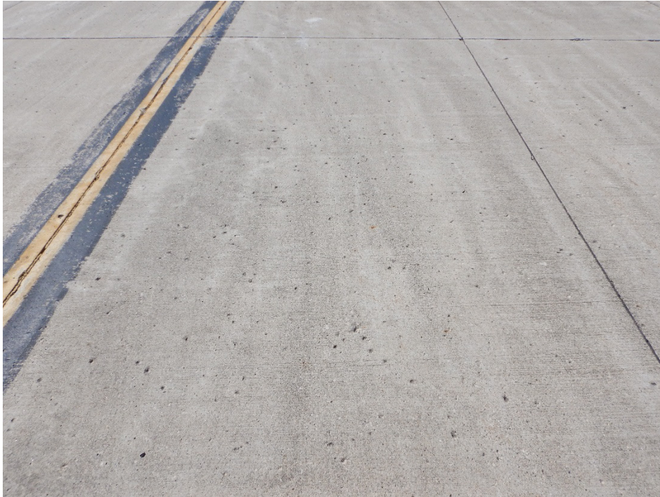
TA4AM-01. Popouts (Sample Unit No. 05).
