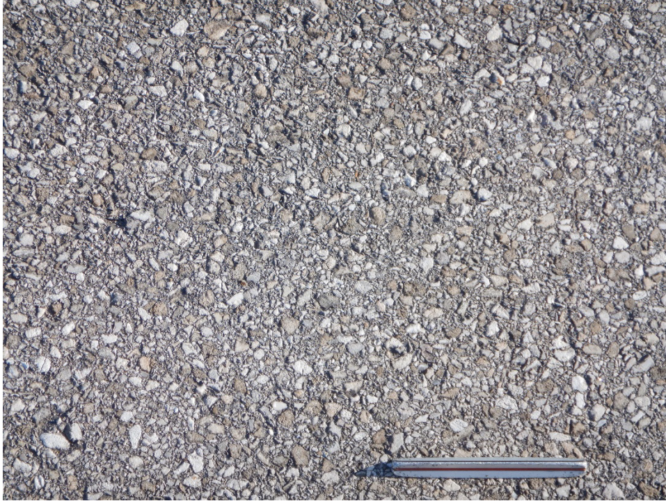
TA2AM-02. Weathering (Sample Unit No. 01).
