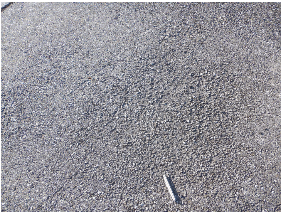
TA2AM-02. Raveling (Sample Unit No. 01).
