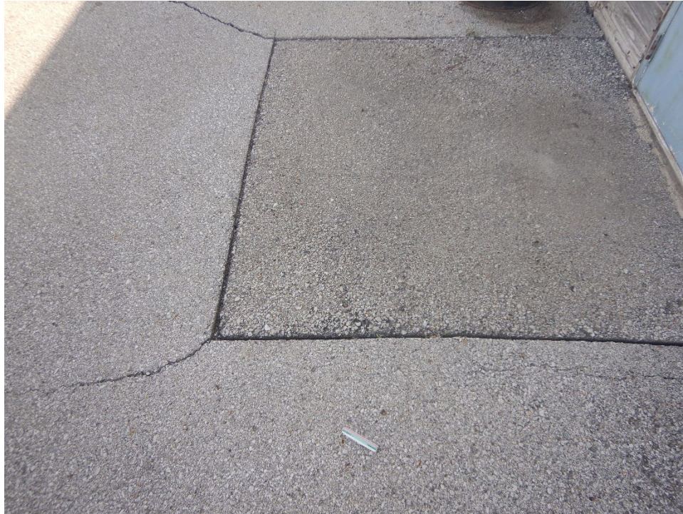
A01AL-03. Patching (Sample Unit No. 01).
