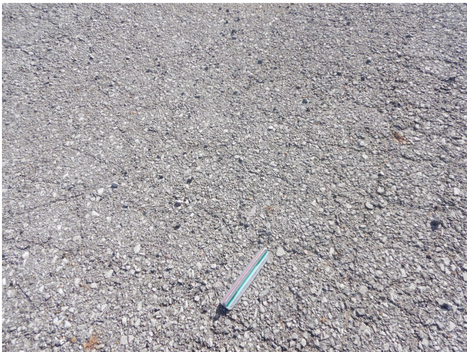
TH01AL-01. Raveling (Sample Unit No. 01).
