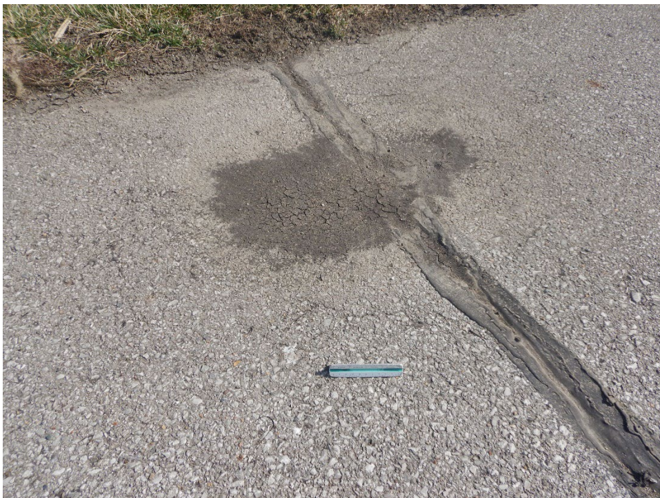
T01AL-01. Depression (Sample Unit No. 01).
