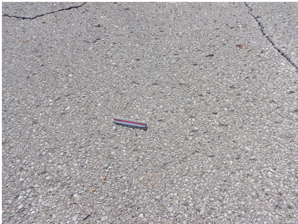
R13AL-02. Raveling (Sample Unit No. 01).
